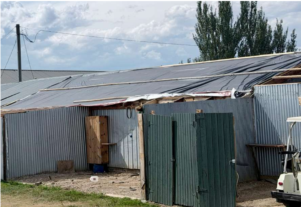
The temporary fix to the roof.
