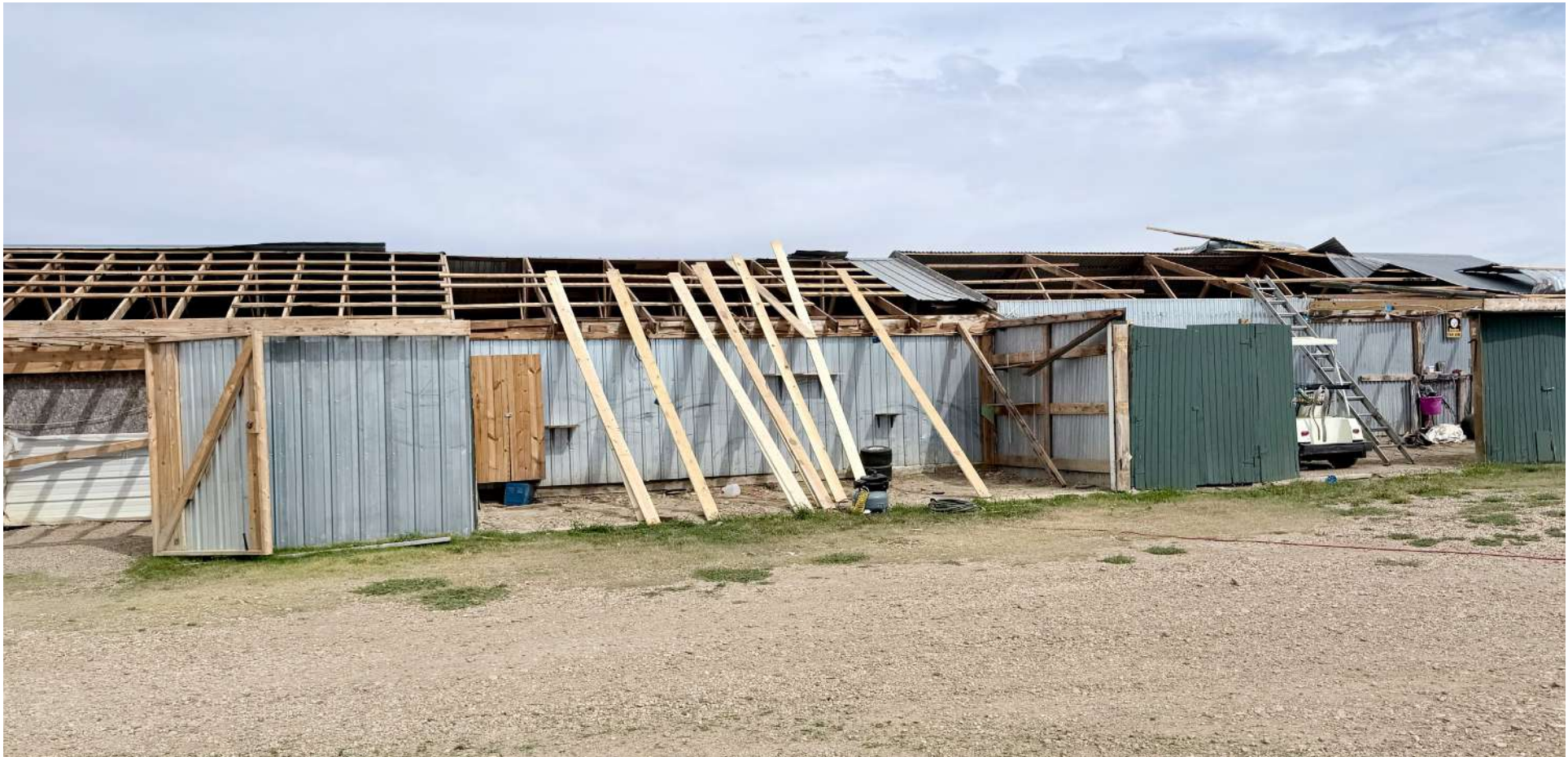
Getting the lumber ready to fix the roof.
