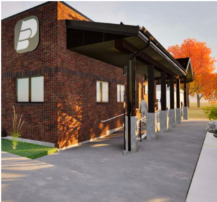
A rendering shows the future Pioneer Trust & Estate Services building, which is expected to open in 2027. Courtesy photo
