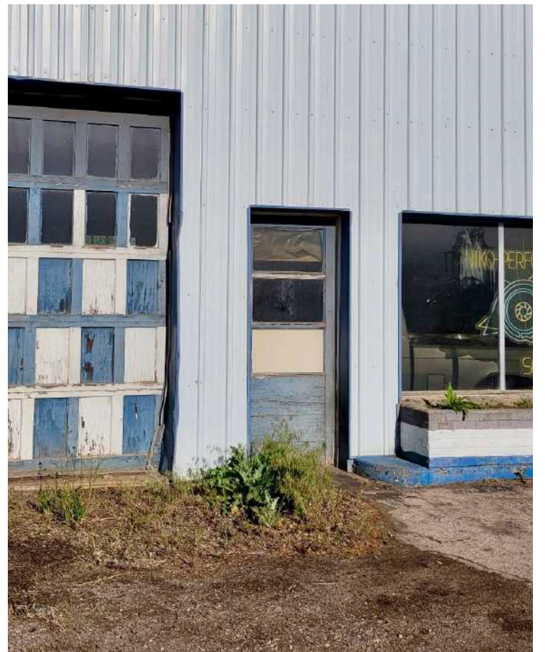
The service station before volunteers began painting and cleaning. Longbrake photos
