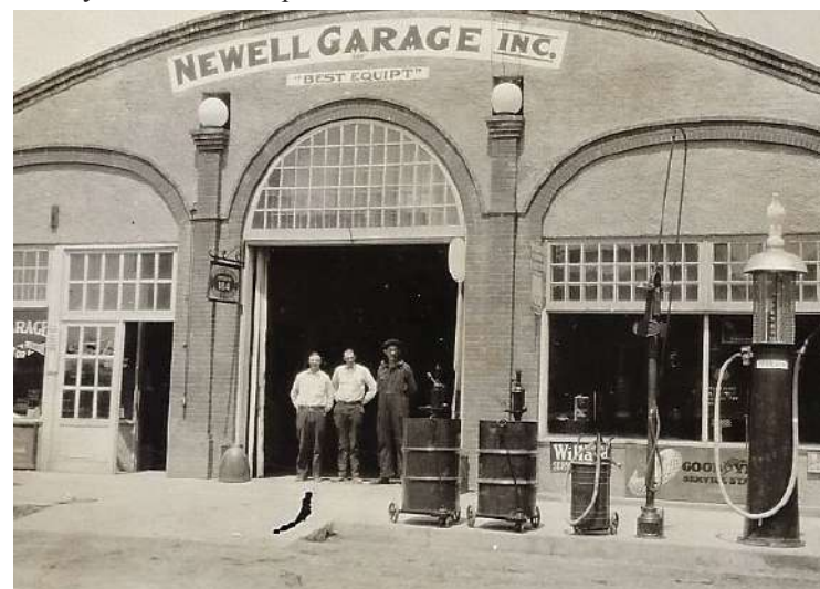
The Newell Garage, now the location of the Newell Museum and Community Hall. Newell Museum
