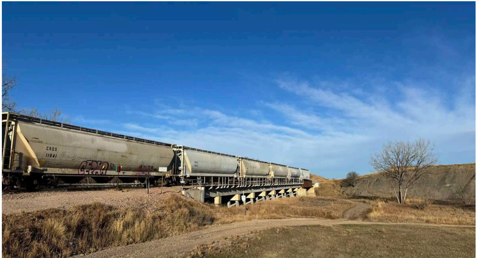
The railroad bridge, west of Masons/Sunny’s
