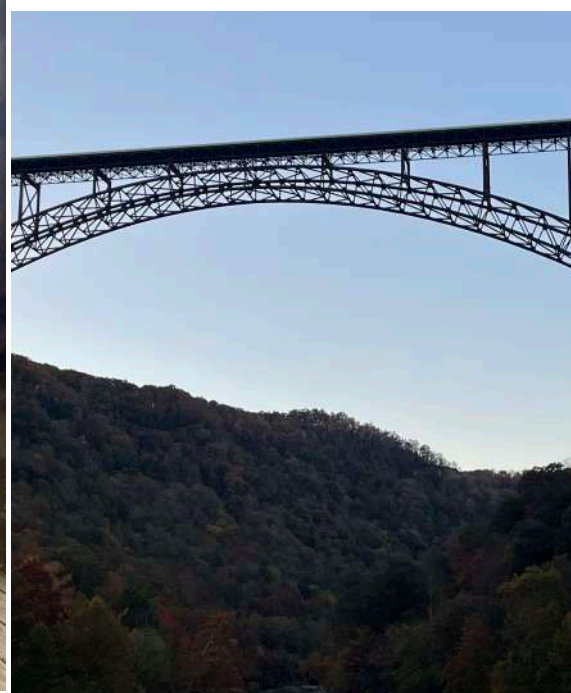
Bridge across the Mountain Valley .
