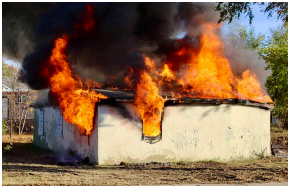
Fire begins to envelop the entire structure.
