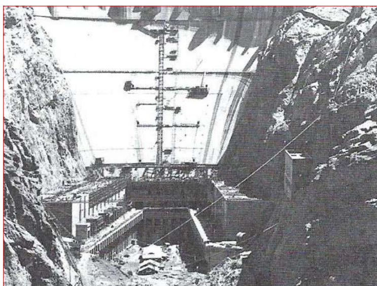
Hoover Dam, (also known as Boulder Dam) under construction. Named for Herbert Hoover, on CO River to control flow, provide irrigation and water supply for Southern CA. Newell Museum
