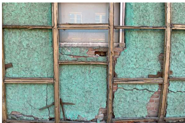
The tin is off the East side of the structure and it uncovered on the building exterior adjacent the structural wall a Brick facade and an exterior stucco layer. (R) 521 State with metal facade removed.
