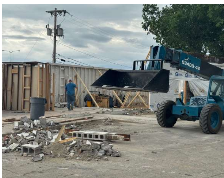
A construction worker turns from demolition clean up to rebuilding and progress on the soon to be “Legends” bank building at corner of 5th & National Streets. Beacon Photo
