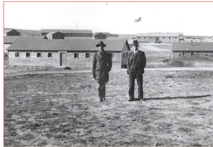
.CCC located at Camp Orman later became Prisoner of War detention center. Camp Superintendent H. B. Gray and F. C. Youngblutt, Manager of Belle Fourche Irrigation Project 1934. Newell Museum photo
