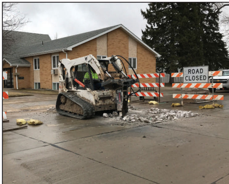
BUSTING UP - Work crews take a pneumatic hammer to the road surface on 8th Avenue near the First Baptist Church last week as scattered concrete panel repair is underway. The procedure is a standard part of new street construction when small cracks can appear in some of the concrete panes. Repair work now saves major problems later. - Beacon Photo
