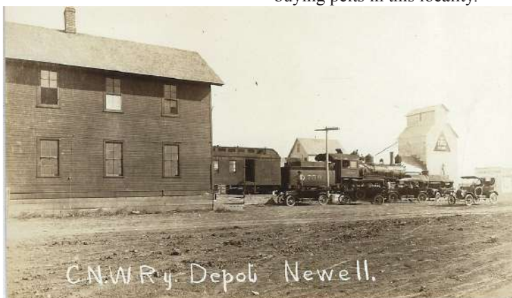
The new elevator was built near the railroad tracks, south of Newell, 1915 Newell Museum
