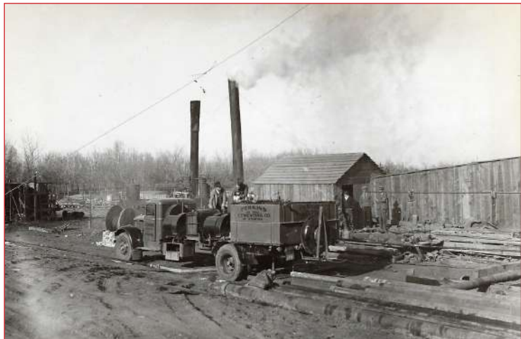
Preparing cement work for drilling the artesian well on the US Experiment Farm. (1933-34) Newell Museum
