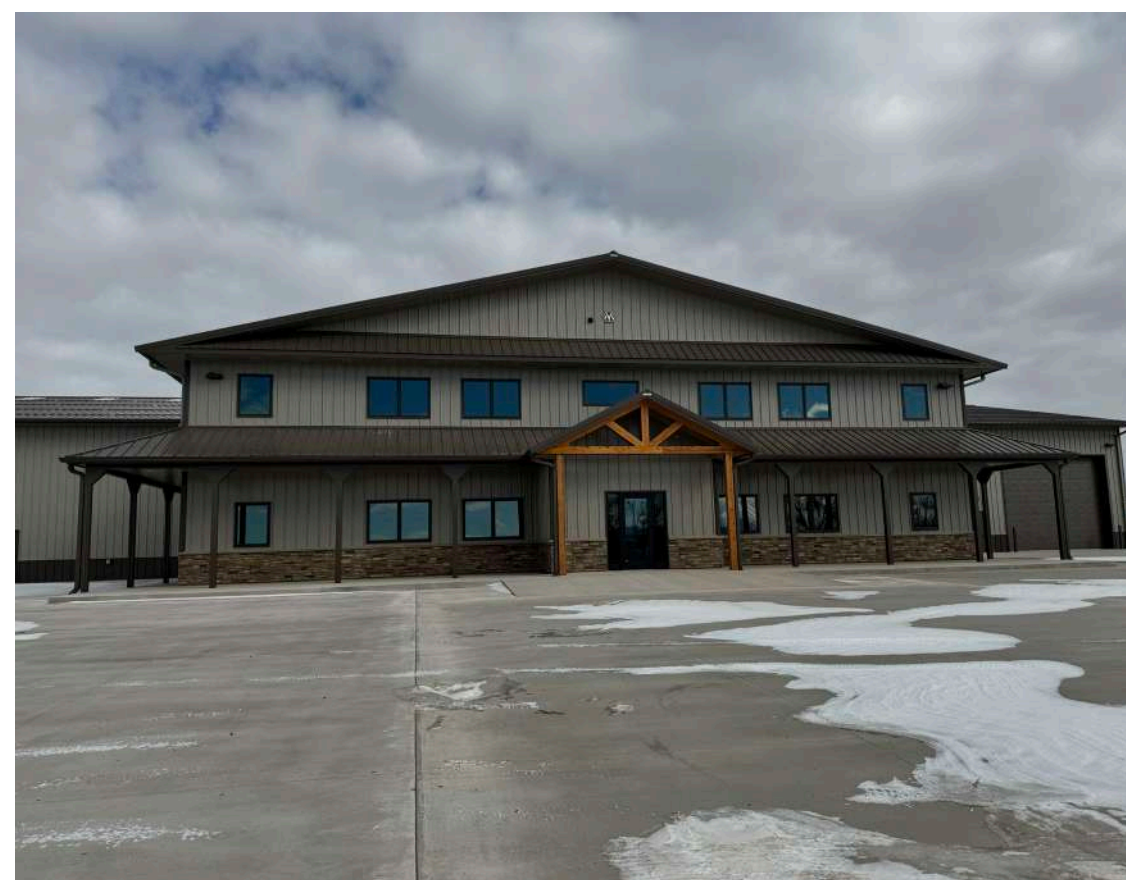
New CBH facility just west of Hwy 212 & 85 intersection.
