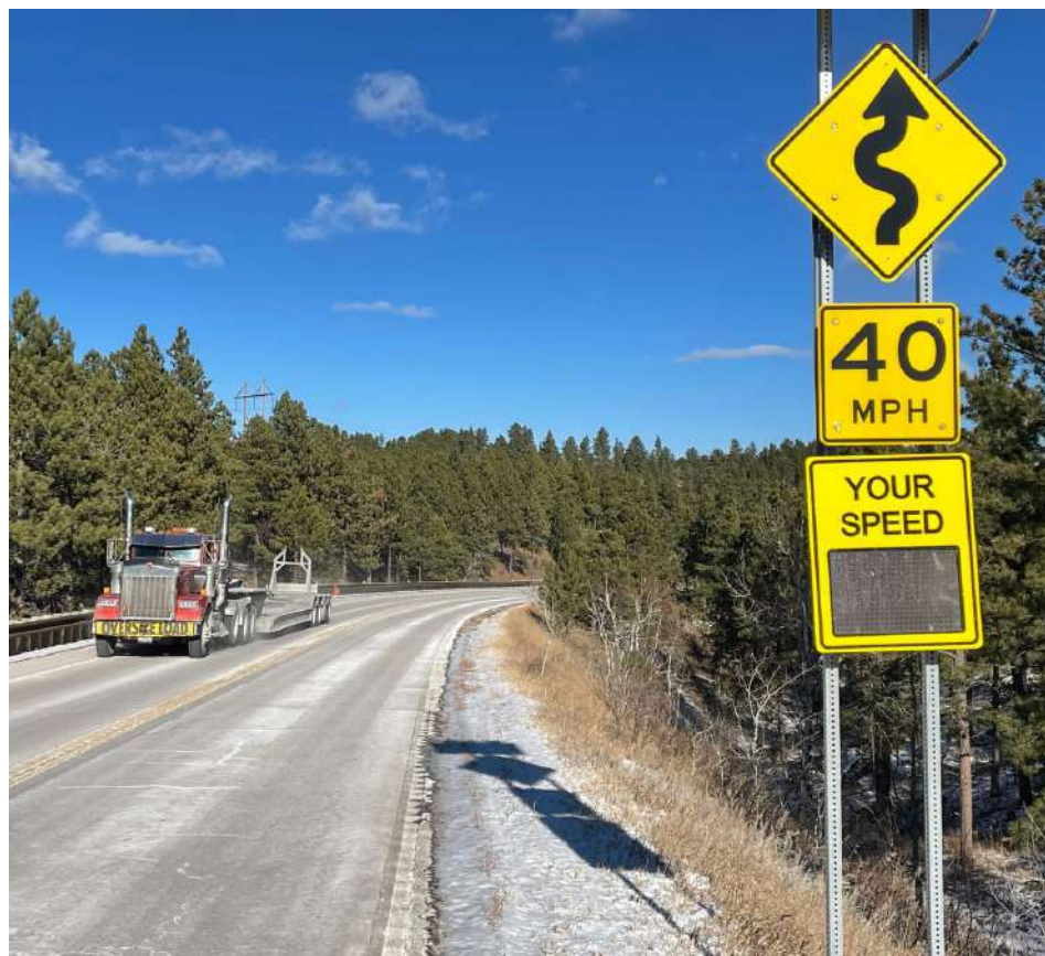
Shoulders are narrow and drop-offs are deep in many locations along U.S. 385 in the central Black Hills, including at this site between Sheridan Lake and Pactola Reservoir. (Photo: Bart Pfankuch / South Dakota News Watch)
