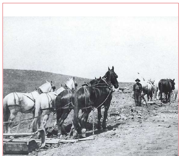
Fresnos in action building the face of Orman Dam 1906 The Ernest Family used this type of equipment to clear snow drifts on roads -Newell Museum
