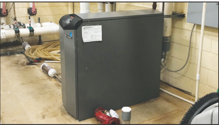
TAKING THE HEAT - The pool water heating unit at the BFACC will be moved upstairs this week away from the pump room where chlorine has begun to degrade the unit.
