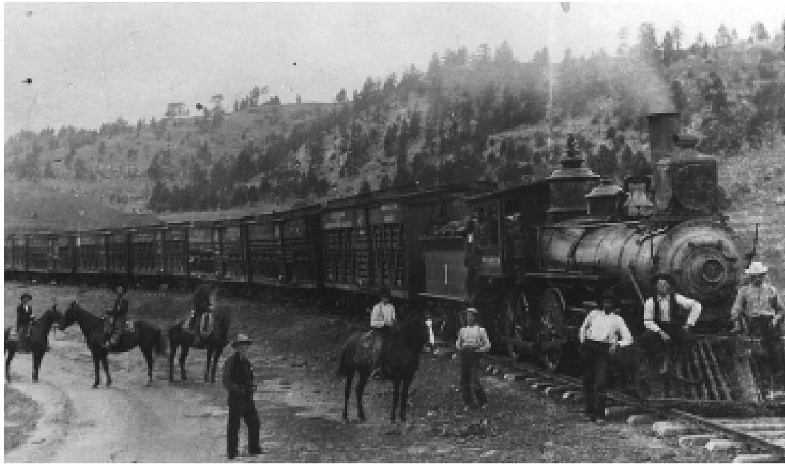
Completed railroad to Hay Creek bridge
