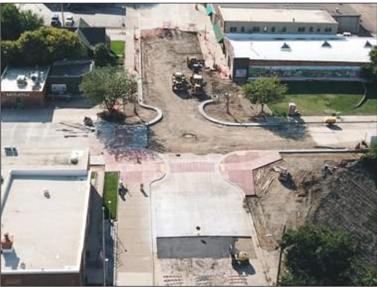
Construction work continues as seen in this aerial view of the intersection of State Street and 8th Avenue. Curb and gutter for the traffic calming "bump outs" is complete and colored concrete installation has begun. Underground infrastructure is complete in the area of the large excavation on State and the hole has been filled in for the most part. Street paving continues on 8th and State.
