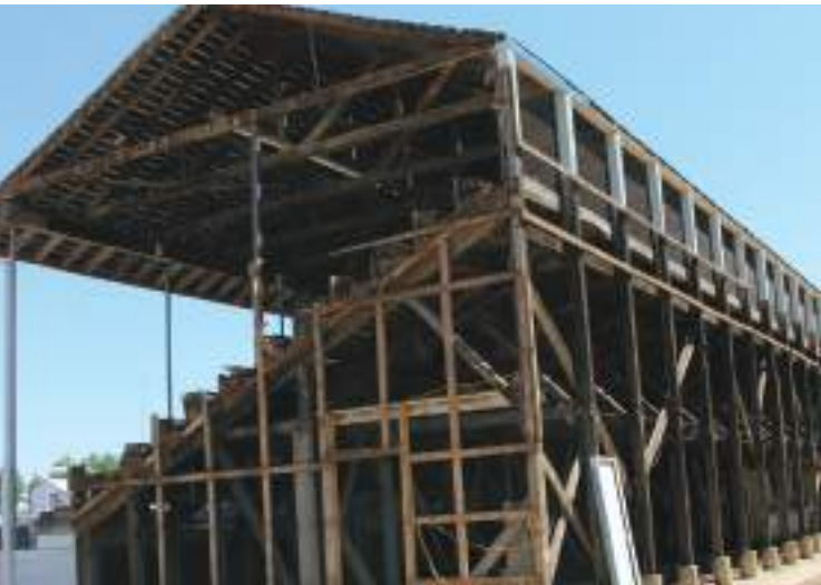
TIN REMOVAL - The first step in the process of demolition of the old grandstands was the removal of the roof and the tin cladding, revealing an infranstructure badly in need of replacement. Photo: Betty Jo Hoffman
