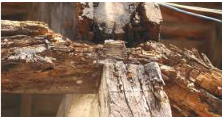
ROTTING AWAY As crews removed the tin cladding on the grandstand the extent of the rotting timbers was revealed.
