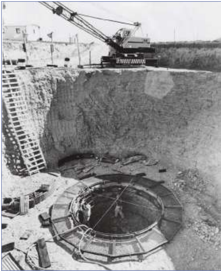
Minute Man (ICBM) site: setting the first lagging plates in place as they begin to excavate the launch tube, which will eventually house the missile
