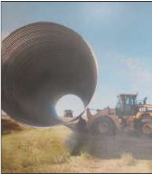
The county highway department recently placed this monstrous culvert at Erk Road, where flood waters had washed the previous one away. -Courtesy photo
