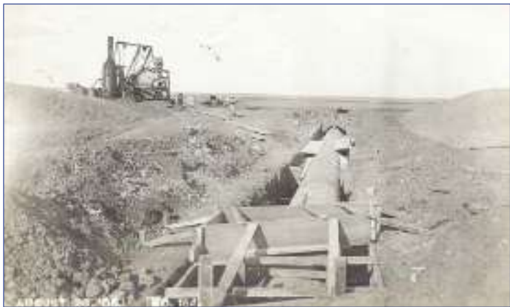
Construction of a flume: used to carry irrigation water over a river or high ground. Circa 1908.
