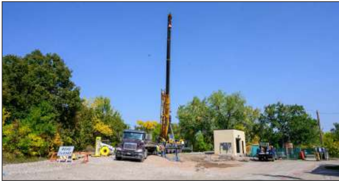
A large crane prepares to lift the back-up generator into place at the new Day Street lift station. The generator is the final piece prior to the new pumps being turned on. The lift station should be operational by Oct. 15th increasing the city’s ability to handle wastewater by 40%. - Hunter Anderson photo
