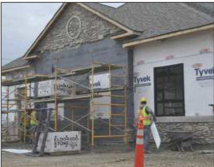
Wilen Masonry is applying the stone work on the Nehl Dental Clinic being built by Ainsworth-Benning Construction. Dr. Nehl is hoping construction will be completed by the end of February.
