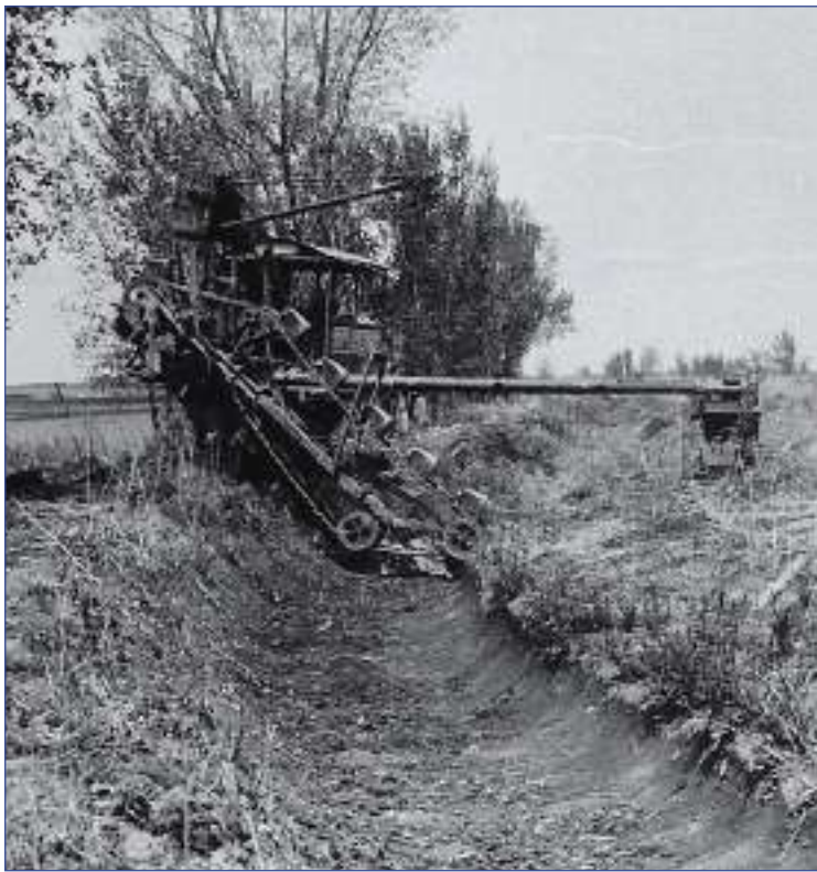
Ruth Dredge - this ladder dredge was used to clean vegetation and silt from ditches, canals and laterals
