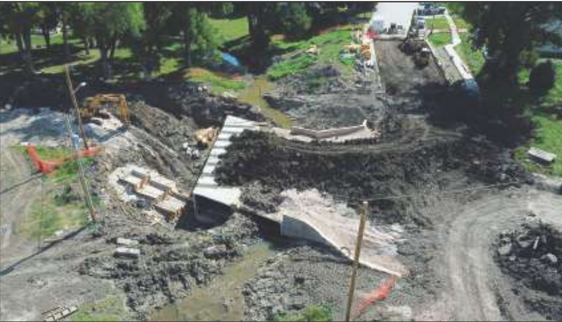
BRIDGING THE GAP - You can see the second box culvert (partially covered with black dirt) now in place as the Hay Creek Bridge moves toward a September completion. In the top right, you can see the work being done on Kingsbury Street and in the right center, the bridge will be tied into 8th Avenue which also has to be rebuilt. The completed wing walls on the south end of the bridge are also visible. Footings for the north end wing walls are also visible (center left). Herrmann Park is in the upper left portion of the photo. -Beacon Photo
