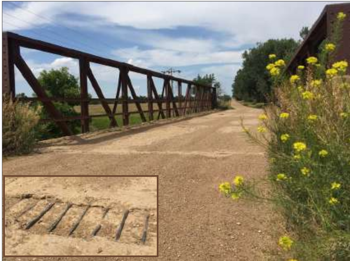
Viken Bridge Closed A state inspection resulted in the closure of two Butte County Bridges, Gaver Bridge and Viken Bridge at the Intersection of Hope Road. Inset shows some of the serious deterioration that exists. -Alexa Althoff Photo
