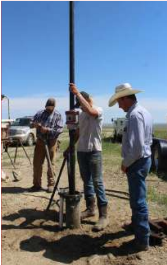
(Left) Matt Mangis, Mangis Construction of Newell, (left) lends a hand as the pump and motor are dropped into the well and fittings are tightened with help from a Keller Drilling employee.. (Right) Matt Mangis, Mangis Construction, who is digging the trunk line in for the Castle Rock Water Corporation, watches as Keller Drilling employees drop in a connector to the tanks that will be filled with water. - Brunner photos
