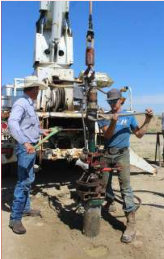
(Left) Matt Mangis, Mangis Construction of Newell, (left) lends a hand as the pump and motor are dropped into the well and fittings are tightened with help from a Keller Drilling employee.. (Right) Matt Mangis, Mangis Construction, who is digging the trunk line in for the Castle Rock Water Corporation, watches as Keller Drilling employees drop in a connector to the tanks that will be filled with water. - Brunner photos
