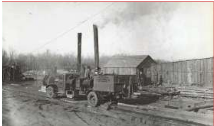
This is a photo of work being done during the drilling of the Artesian well at the Experiment Farm. This photo is of cement equipment being used. The markings on the side of the mixer read “Perkins Oil & Well Cementing Co. of Wyoming.”
