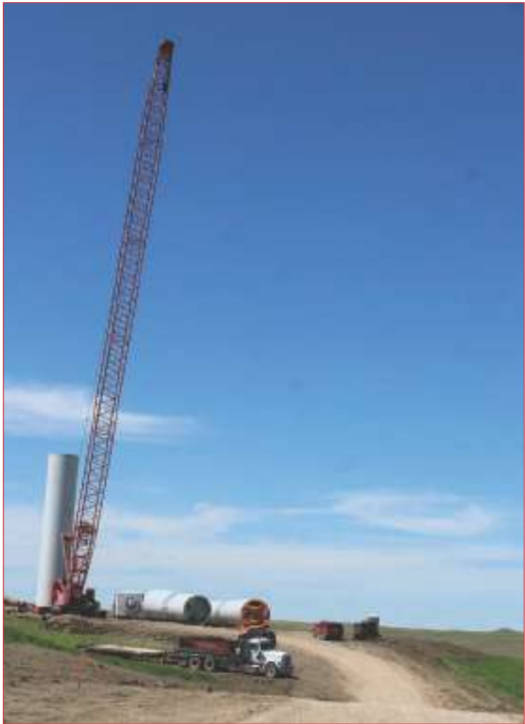
GOING UP - Large cranes break up the skyline on the prairie as they lift the individual sections of each wind turbine tower into place at the Willow Creek Windfarm project, located northeast of Newell. - Brunner photo
