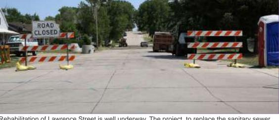
Rehabilitation of Lawrence Street is well underway. The project, to replace the sanitary sewer lines, other underground infrastructure and resurfacing will cost just under \$1 million. A&L Contractors of Spearfish is the general contractor. - Beacon Photo
