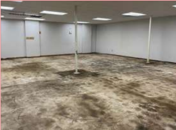
All the flooring material has been removed in the high school weight room and its ready to be prepped for the new interlocking rubber floor mats. - Brunner photo
