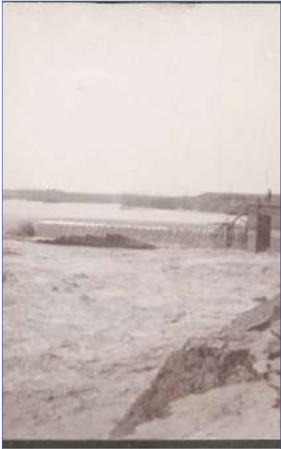
Heavy spring flooding breeches the diversion dam.
