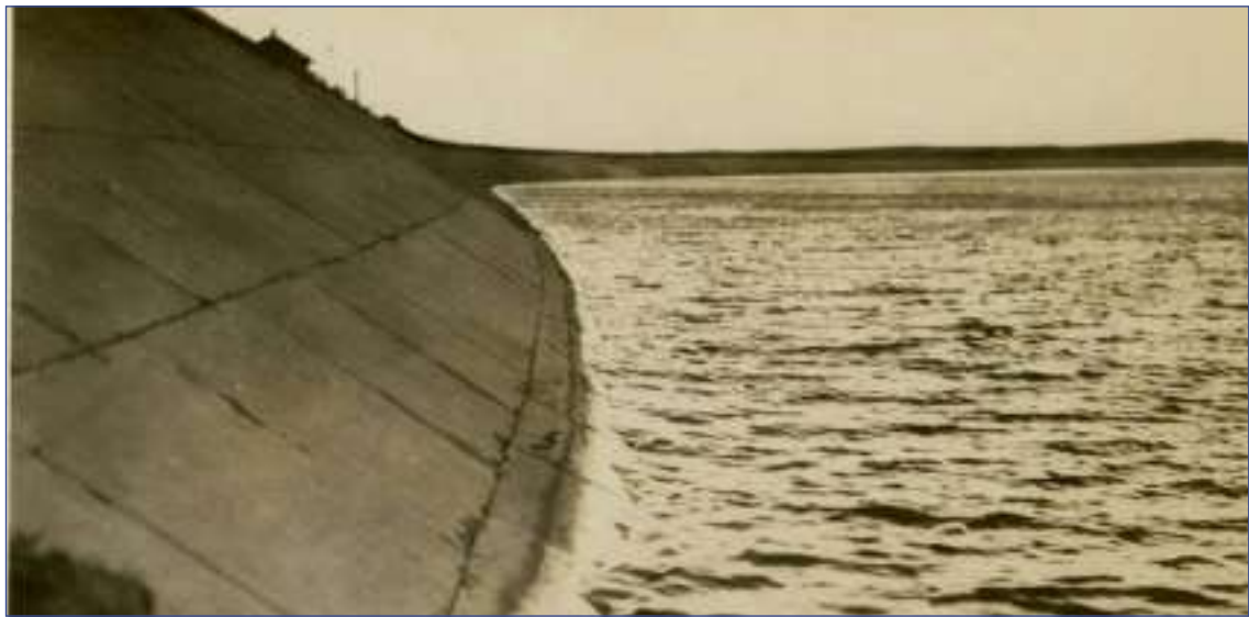
The face of the Orman Dam where the concrete blocks are visible.
