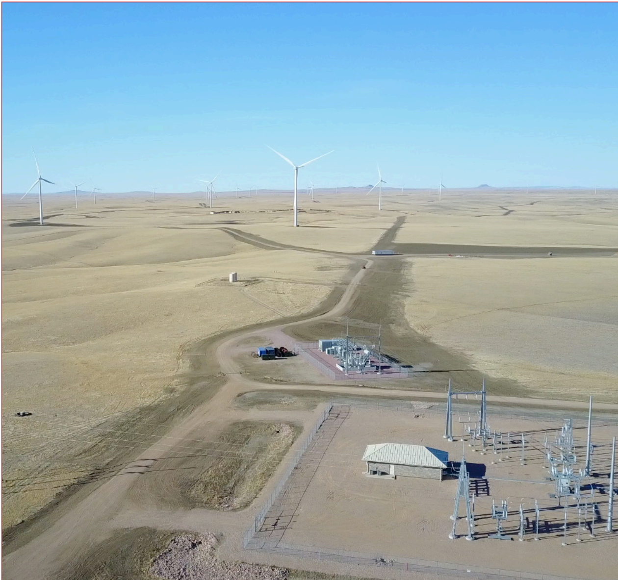
An aerial view of the Willow Creek Wind Farm northeast of Newell. The facility has a 103-megawatt (MW) capacity consisting of approximately 45 wind turbines, associated access roads, a new collector substation, an operations and maintenance facility, temporary staging areas, and associated transmission interconnection facilities. - Beacon photo
