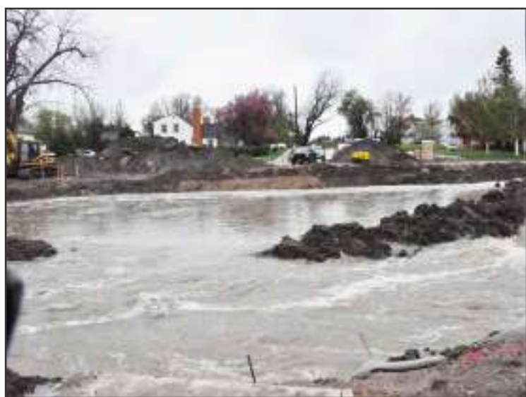
FLOODED - High water on Hay Creek damaged construction work on the new 8th Ave. crossing. The diversion wall was breached flooding the first culvert and it's footing. It's unknown if work can be completed by July 4th. - Beacon Photo
