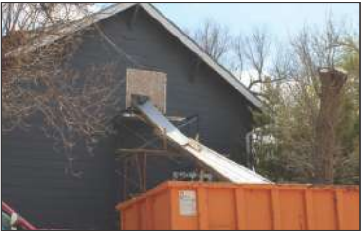
CHUTE! - Komes Construction is already busy tearing out smoke and water damaged walls, ceilings and insulation. Todd set up this handy slide so they didn’t have to carry the damaged materials downstairs. -Brunner photo
