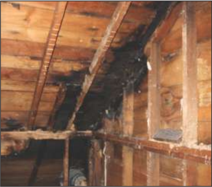
This is the only fire damage that the couple could see on the inside of their home. However there is significant damage around the chimney area and roof, as well as smoke and water damage. -Brunner photo
