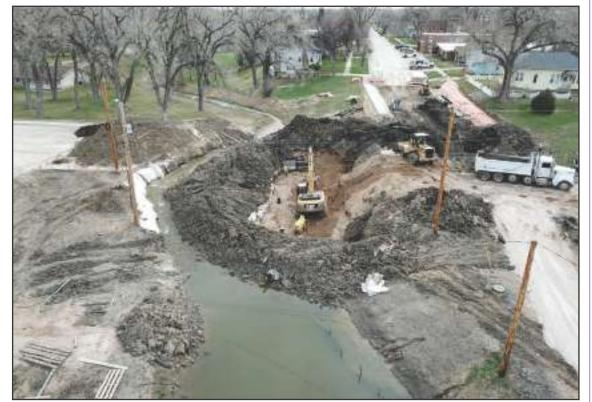
**MAKING HAY (CREEK BRIDGE) WHILE THE SUN SHINES -** Work crews from Ainsworth -Benning Construction are making good progress on the new 8th Avenue Hay Creek Bridge. As can be seen above, a diversion in the water-flow has been created to allow excavators (center) to build the foundation for the new box culverts. *-Beacon photo*
