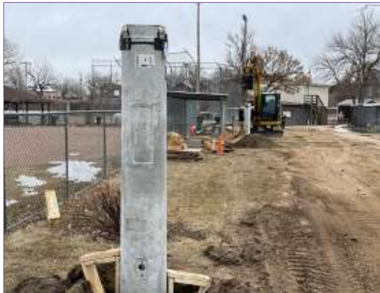
Concrete pillars are popping up at the Roundup Sports Complex where new lighting poles will be installed. Crews from 21 Electric in Newcastle, WY, are working with Musco Lighting on the installation. There will be 26 pillars placed around the six ball fields. The 60-foot high LED light standards will slip over the concrete pillars and be able to withstand 100-mph winds. Beacon Photo
