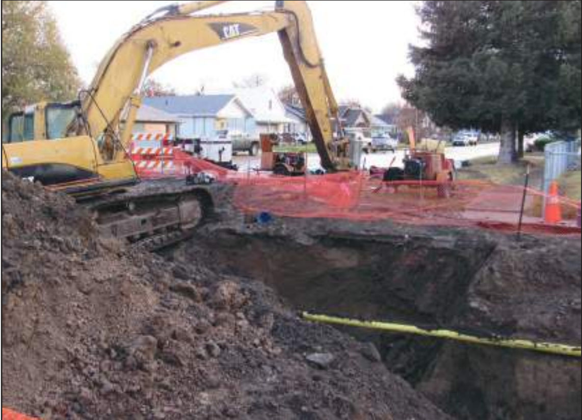
Excavation at 8th Ave. and Lawrence Street. Last sewer hole to fill in before crossing Hay Creek. Exposed new MDU line (yellow)
