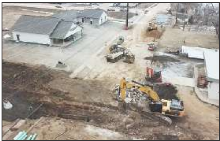
DIGGING AWAY - A 20-foot deep trench (foreground) bisects National Street where the new sewer line will go. Paving on National Street over the Hay Creek culvert is also underway (top center-left of photo). Crews lost a day to the weather last week and this week as well. - BF Beacon photo
