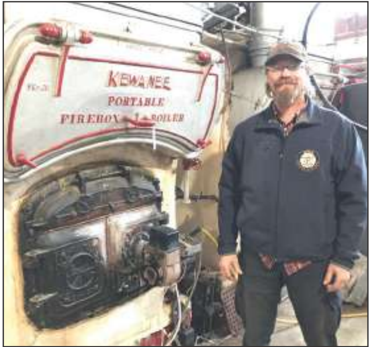
WELL "OILED" BOILER - Building owner James Pietila stands next to one of the two original massive boilers that heat the Roosevelt Center. In the 1920's they required 500 pounds of coal daily on a 10-degree day to heat the school. Today he's converted this boiler to burn waste oil, primarily the oil from cars and trucks after an oil change. Pietila gets the oil locally, the majority of it from Hersurd's. - Beacon photo
