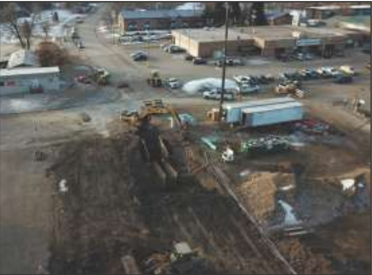
DIGGING IN - Construction crews are preparing to dig the trenches for the new sewer main under National Street. The installation should take place this week with repaving of National Street from here over the Hay Creek culvert to take place next week. -Beacon Photo
